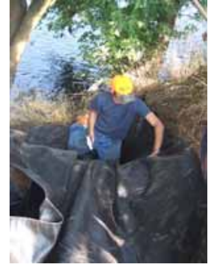
Geotextile fabric being laid down.
